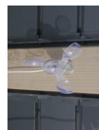
9. (optional) Position the various sensors (rain, temperature and wind) on the pergola structure. Ensure that they are sufficiently exposed to detect the climatic variations required.
