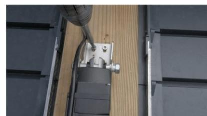
**4. (Bis)** Fix the jack support to the structure, making sure that the slats of the pergola are always closed.
