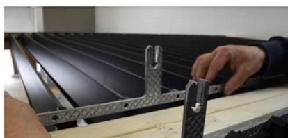
**1.** Replace the rods with the forks by clipping them into the blade holders. Position them from the second set. Lock the assembly with the latches.
