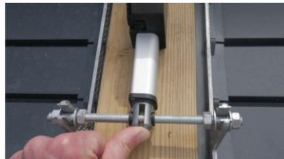
**4.** Press lightly on the cylinder or forks so that they are fully closed before fixing the bracket.
