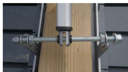
**3.** Manually close the slats of the pergola and insert the fork pin on the two metal rods.
