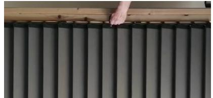
8. Check the movement of the stopper by rotating it. It is finished!
