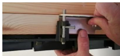
5. When the kits are in the closed position, place the plate on the edge of the post, so that the lock fits into the top hole.
