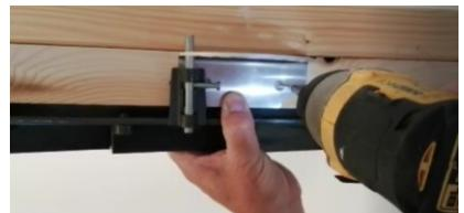
6. Check that the lock fits into each of the holes and screw the plate onto the post.
