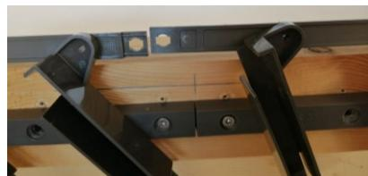
1. The SAM kit should be fixed 15mm from the edge of the post (use the PVC joint bar as a template).
