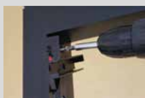
Tighten screw until snug
